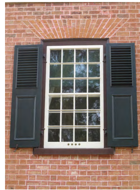
Window restoration at the Wissler-Cascaden House showing the reflective quality of the historic glass. Source: Ron and Wendy Cascaden
